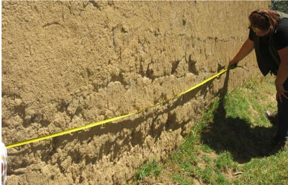
Figura 42. CM-04 BASE EROSIONADA
