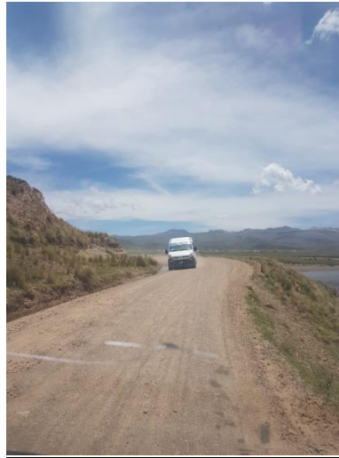
Tramo: Vila Vila-Chivay, km06+100
